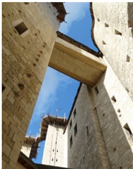
The Church of St. Francis and St. Clare. From the archives of Municipal Office in Tychy
